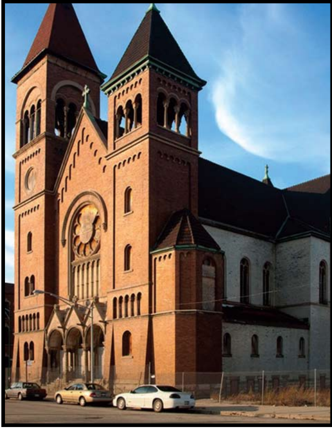
St. Boniface Church Noble and Chestnut Street Architect: Henry J. Schlacks
