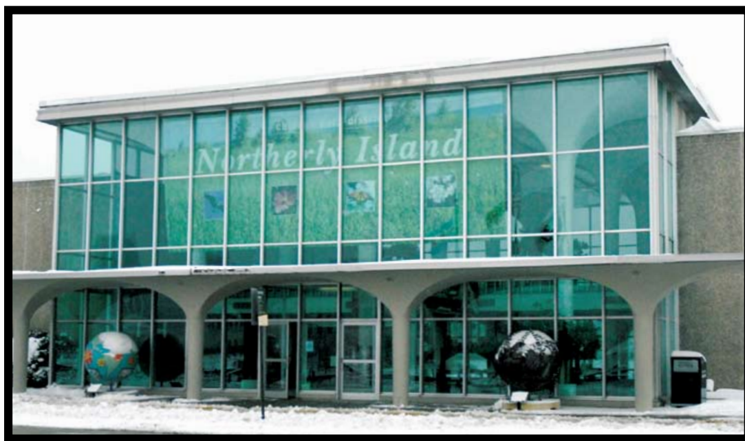
Meigs Field Terminal Northerly Island Architect: Consoer & Morgan
