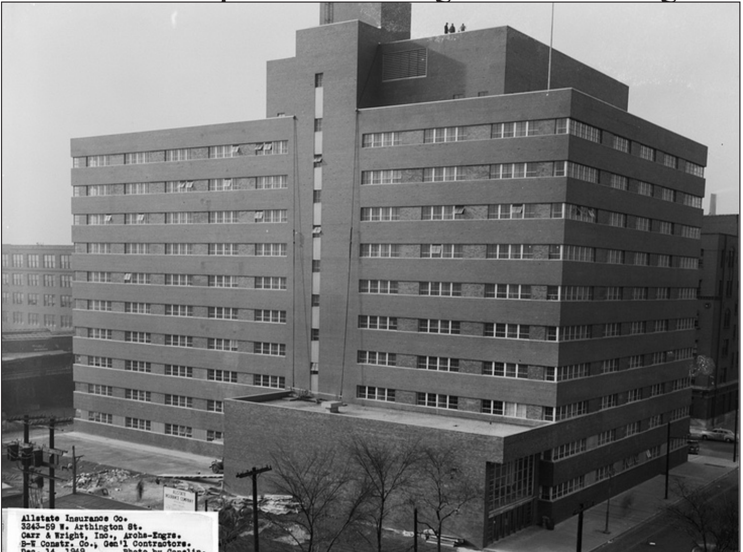
Allstate Building, Photo Credit: Jacob Kaplan
